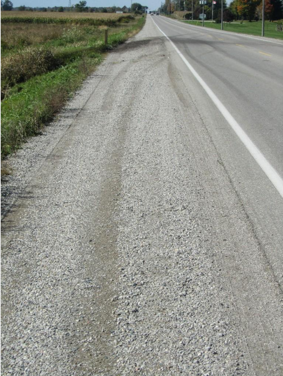
View, looking west along the south shoulder of the Medway Road and showing yaw marks in the gravel caused by the deceased's vehicle as it rotated clockwise and curved back onto the paved road surface.
