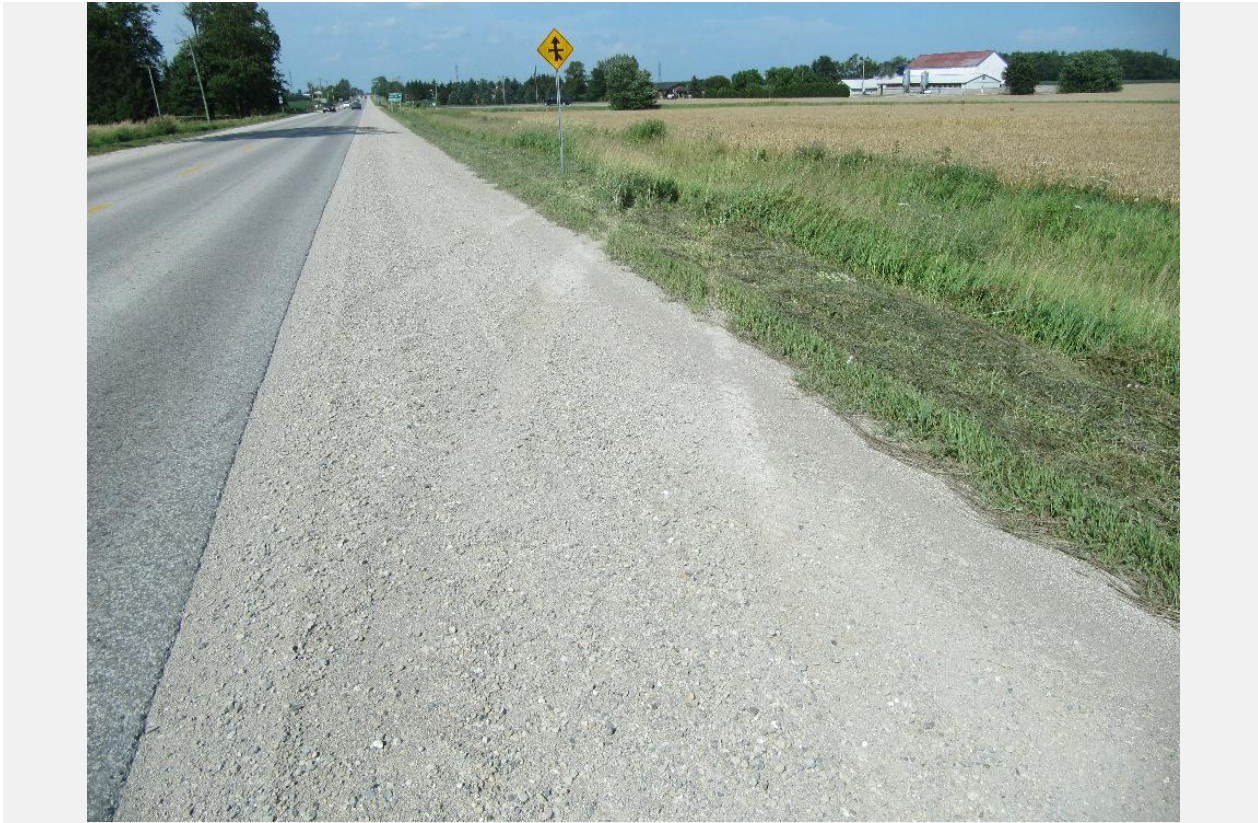
Loss-of-control tire marks on a freshly re-graded gravel shoulder leading to a rollover in grassy roadside of a rural highway.
